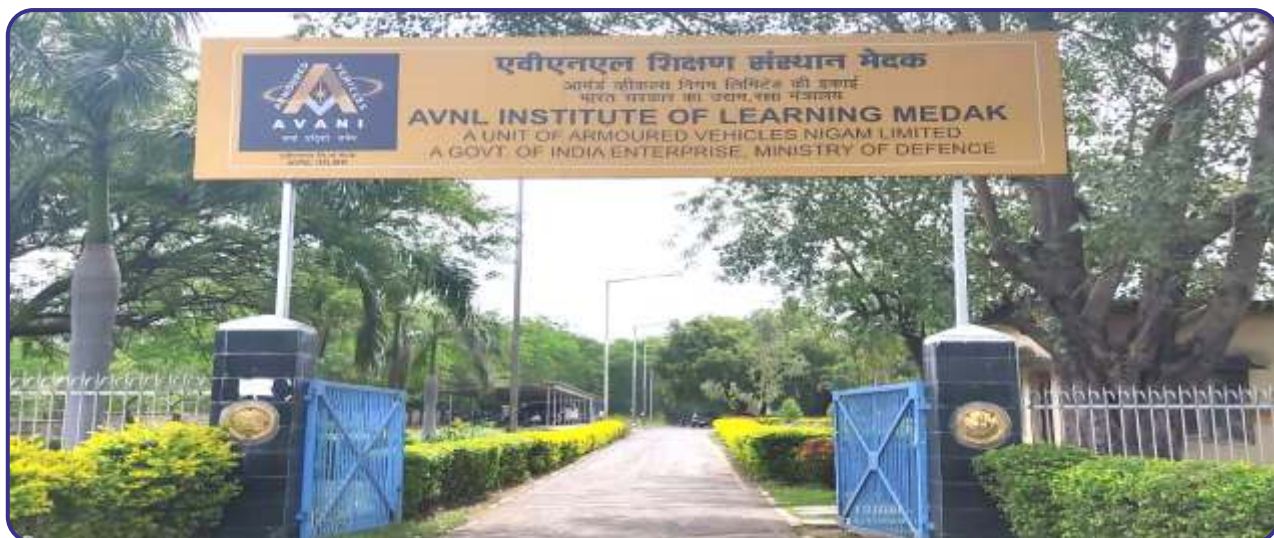
AVNL IOLMK OFFICE BUILDING
